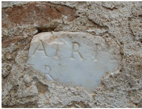
Figure 1.2: Ancient Stonework Used in “New Build” Walls [1.1]
