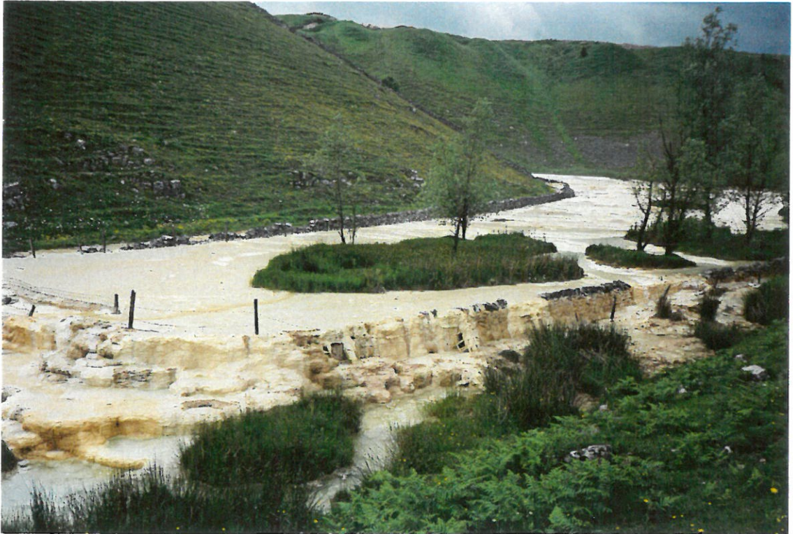
Plate A2.11: Lime ash tips, visible in the background of the photograph.
