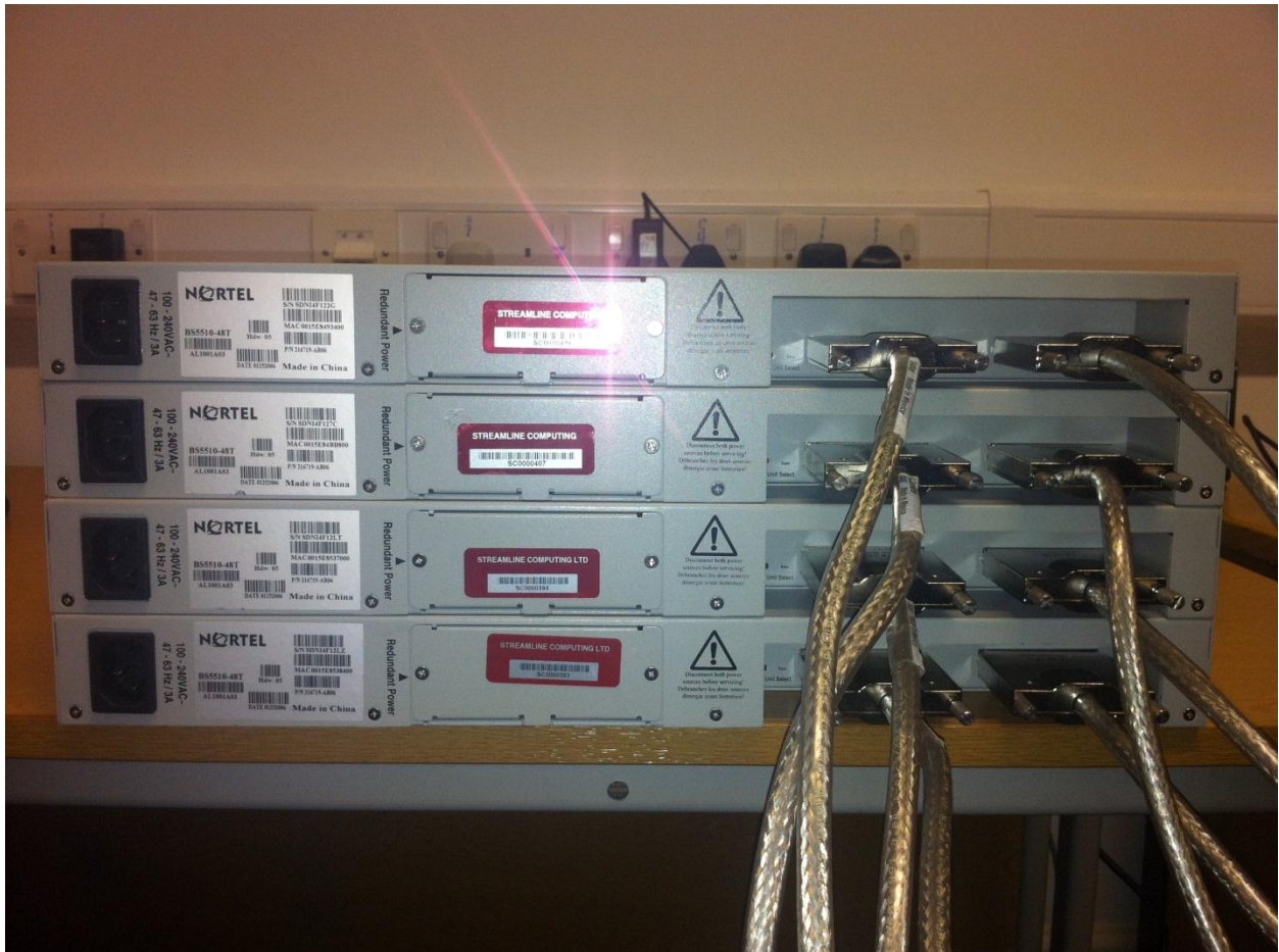
Figure 16: Nortel Baystack 5510-T Layer 3 Switch
