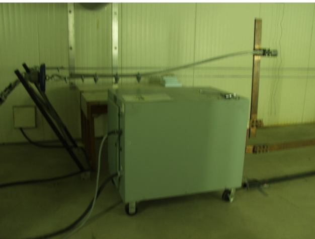
Fig. 2. The generator and its connection to the cable
